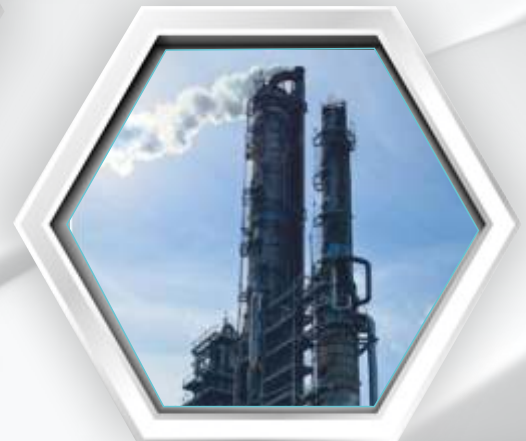
PETROCHEMICAL & REFINERY INDUSTRY
